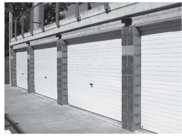
Tongue and groove panel profile, 0.6mm, roll formed Colorbond G2NS steel. Five wide ribs across each panel, in a shiplap board effect.
